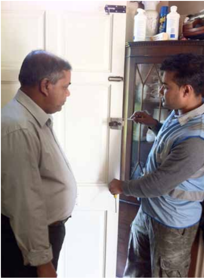
Contractor carrying out repair work
